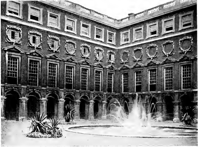
189. Fountain Court, Hampton Court Palace.
